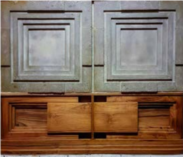
Typical Wall dado This involves crafting cast-in-place concrete tiles using custom-made silicon moulds, complemented by solid wood tiles designed to specification.
